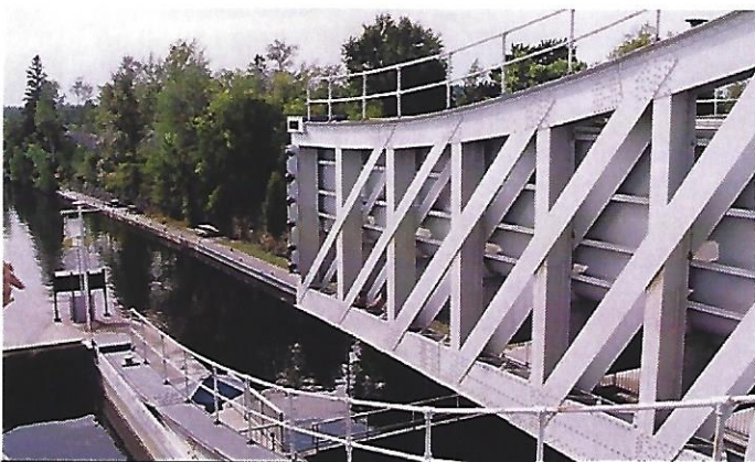
Constructed between 1896 and 1907, the Kirkfield Liftlock closely resembles the Peterborough Liftlock. Each pan holds 228,093 gallons of water weighing 1,700 tons, except that one foot of water weighing 144 tons is added to the upper pan to make it heavier than the lower one. This imbalance is the basis of lock operation.
